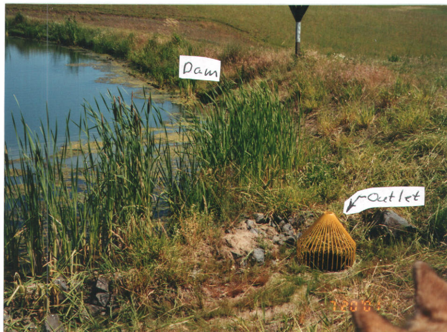
Photo 2. Showing Pond Outlet.
