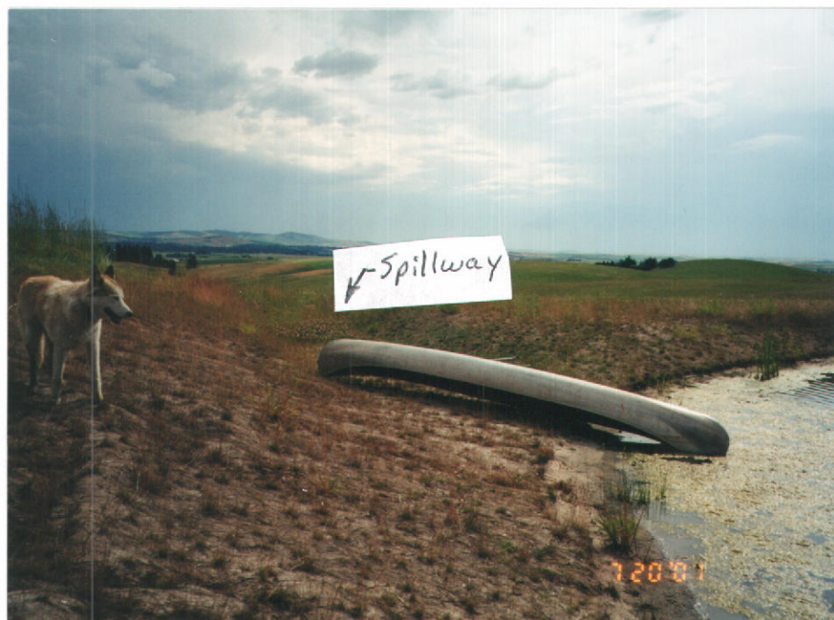
Photo 3. Showing Emergency Spillway.
