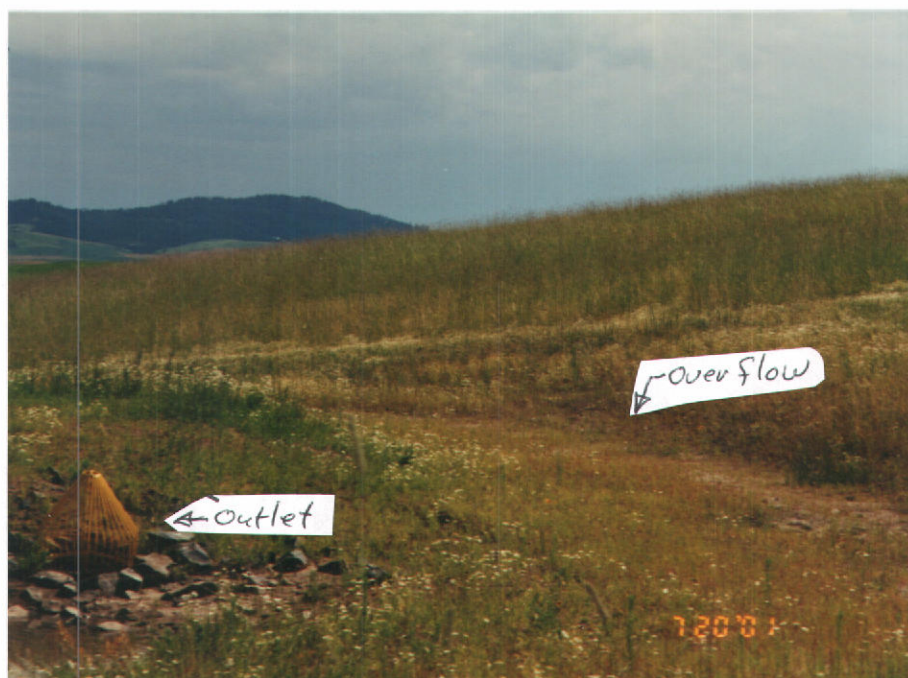
Photo 2. Showing Emergency Overflow.
