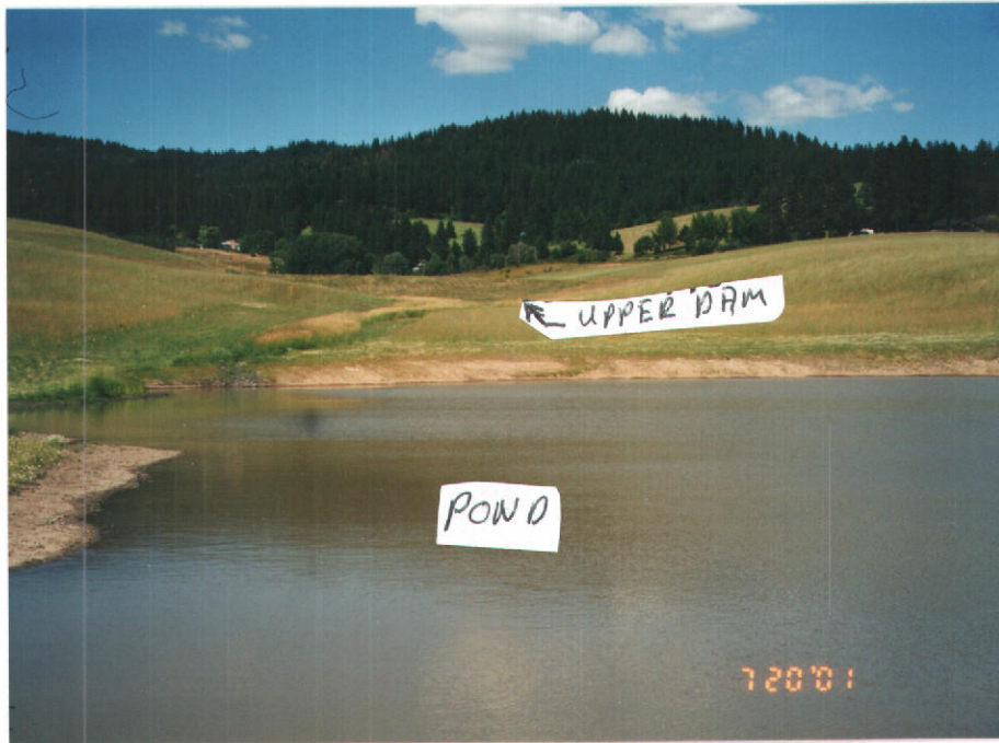
Photo 3. Showing Pond (87-07217) in Direction of Upper Pond (87-07216).
