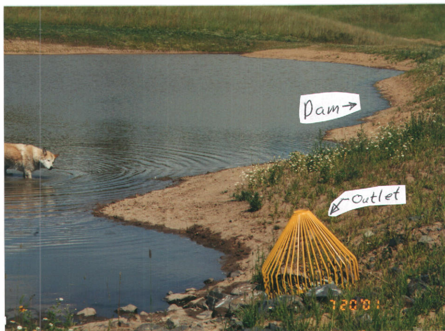
Photo 1. Showing Pond Outlet.
