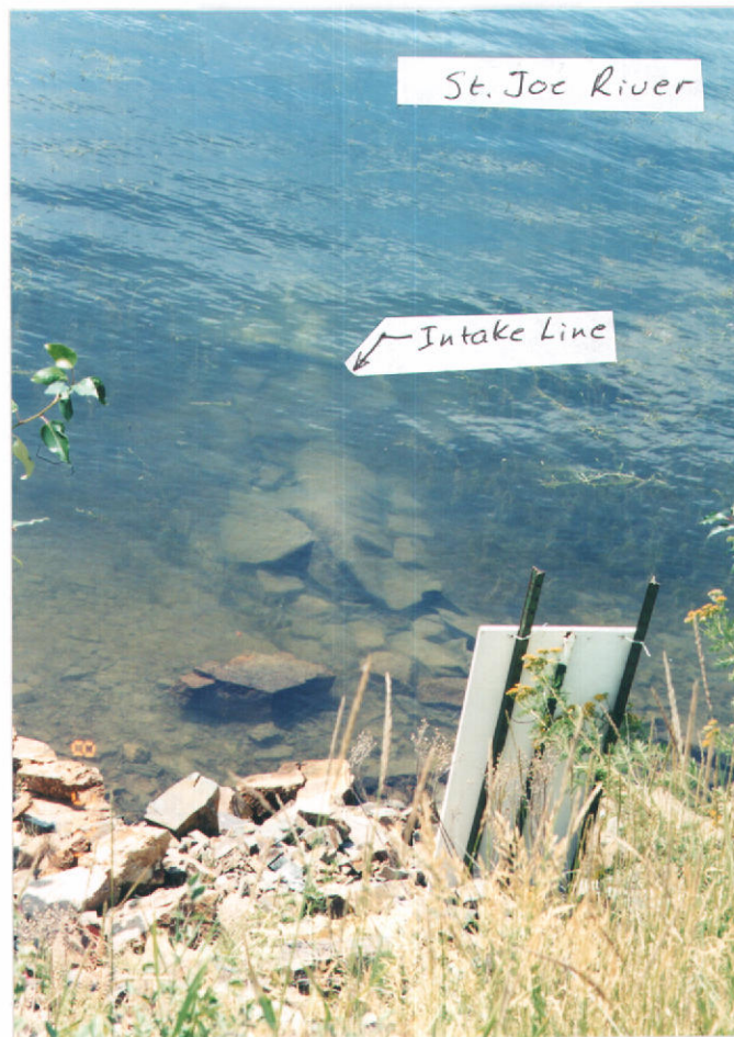
Photo 1. Showing Point of Diversion (POD).
