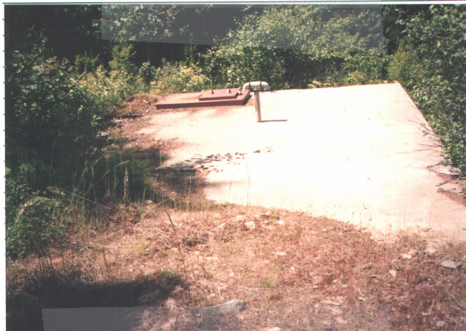
CONCRETE STORAGE TANK & LOOKING N. WESTERLY
