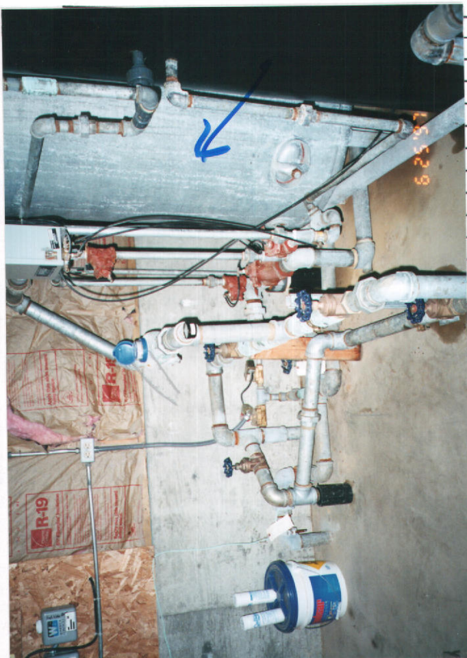
WATER SOFTENER & FLOWMETER FOR WELL #1 AND TOTAL SYSTEM* WELL HOUSE & STORAGE TANKS
