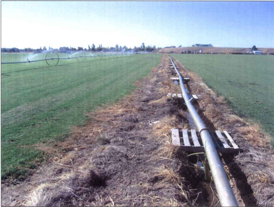
Photo 3: Taken at northern end of field facing towards mainline bend shown in Photo 2. Place of use is east (left) of aluminum mainline.
