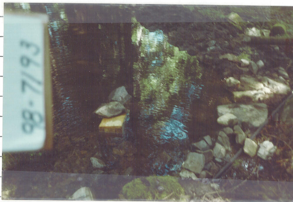
POINT OF DIVERSION
