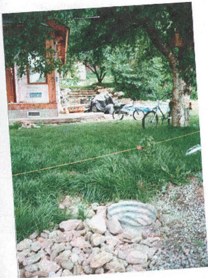
PICTURE TAKEN FROM CO. RD. FACING WEST. ACCESS CMP TO BURIED CULVERT UNDER CO. RD.
