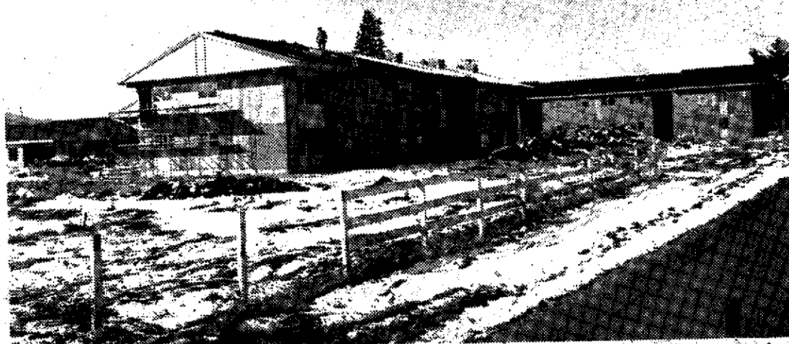
Three Multi-unit Apartment Buildings are being brought to completion on Division Ave. east of the New Farmin school. The development takes up the frontage from Spruce to Hickory. Collins Construction is building the apartments which will take up some of the demand for rental housing. — N-B photo.
