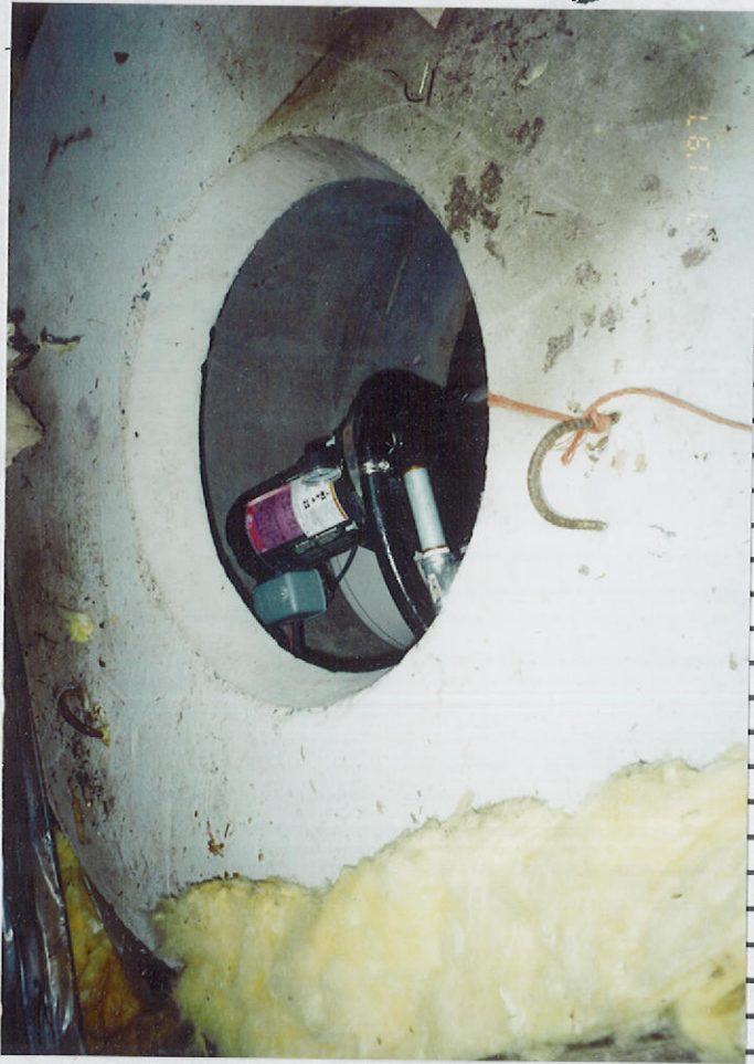
STATE OF IDAHO DEPARTMENT OF WATER REPORT SUPERVISOR GEOGRAPHIC 1/2 HP Craftsman Pump w/ Pressure Tank
