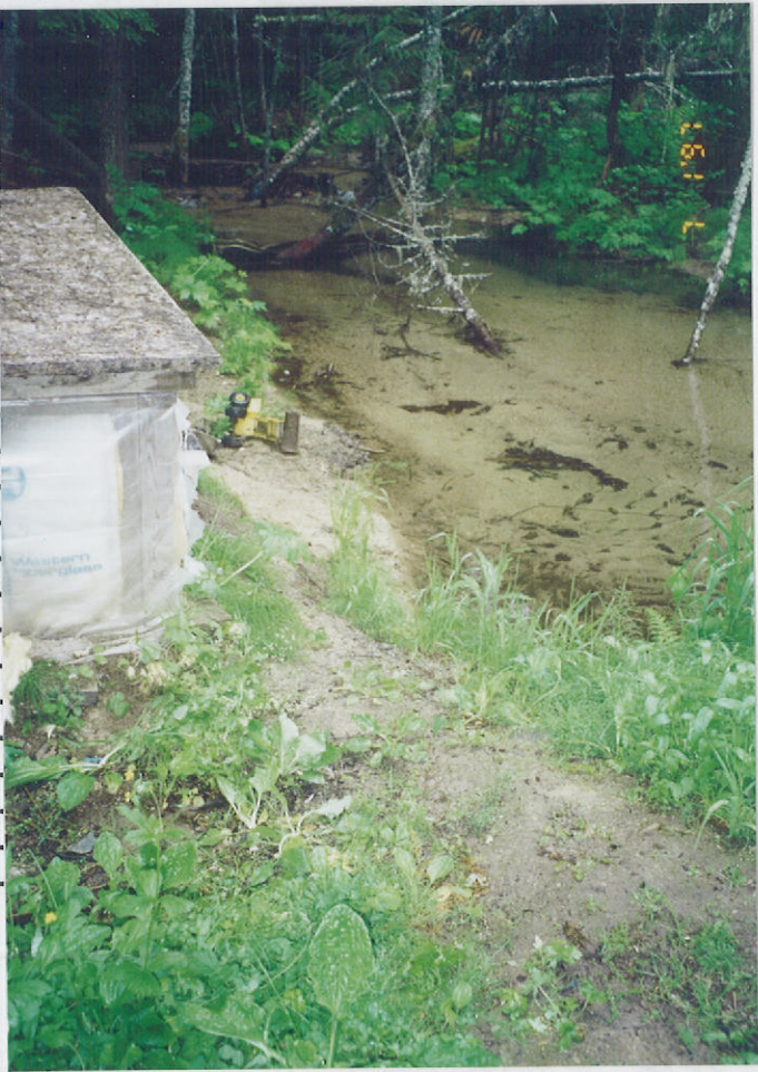
Slotted Concrete Cistern next to Creek for Infiltration & Pump Location
