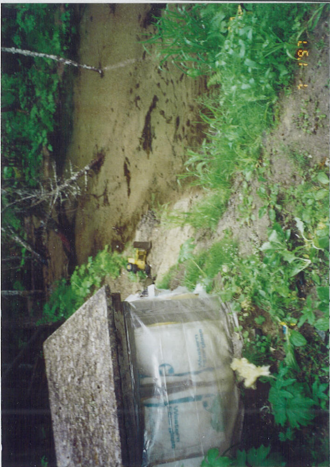
Slotted Concrete Cistern next to Creek for Infiltration & Pump Location
