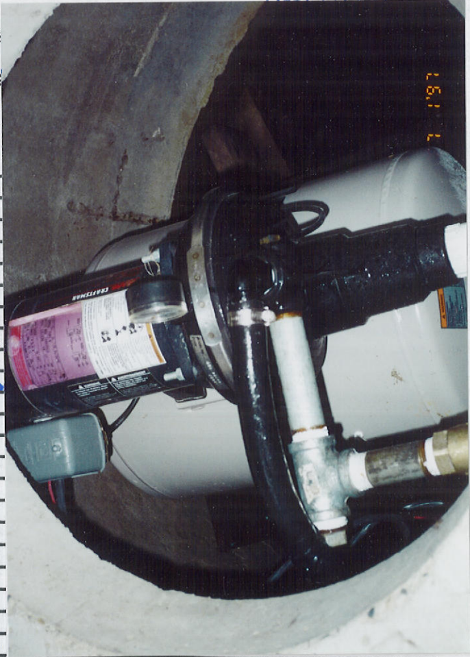
STATE OF IDAHO DEPARTMENT OF WATER REPORT SUPERVISOR GEOGRAPHIC 1/2 HP Craftsman Pump w/ Pressure Tank
