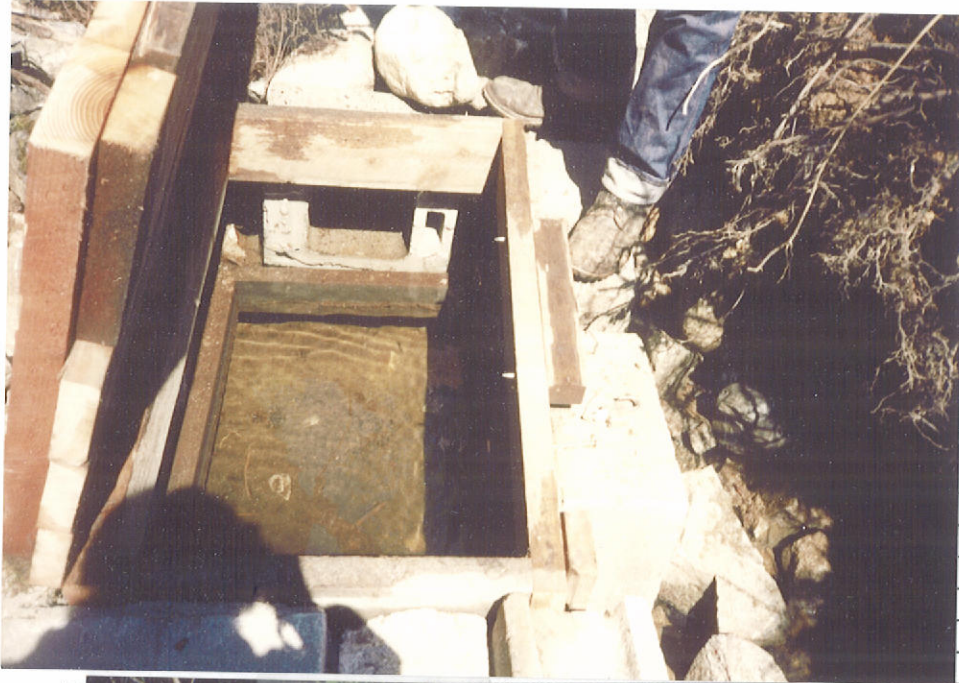
Point of Diversion
