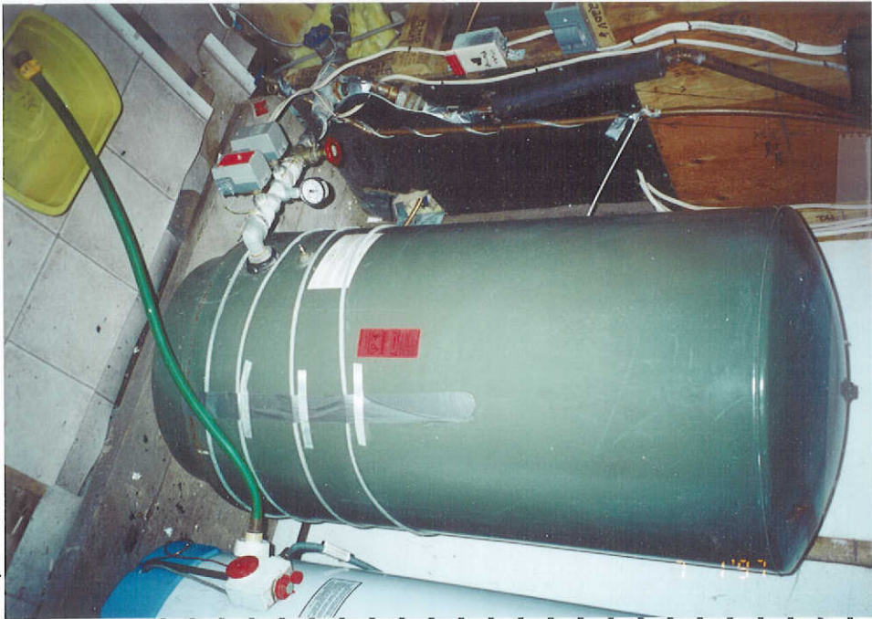
Pressure Tank on Back of House Cistern
