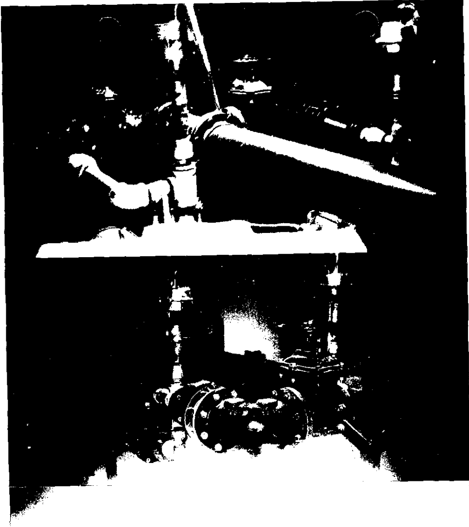
Pumping Station from storage to IRR Sys.
