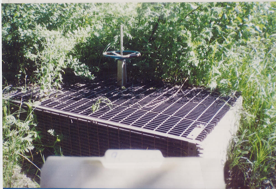
INTAKE AT GROUSE CREEK
