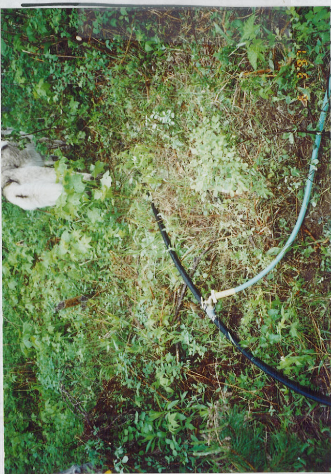
1" BLACK PVC PIPE DISCHARGE GARDEN AREA
