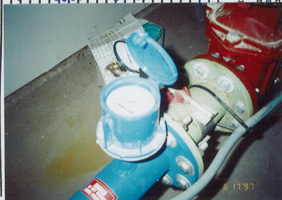
Valves in Pump House McCombs Flowmeter
