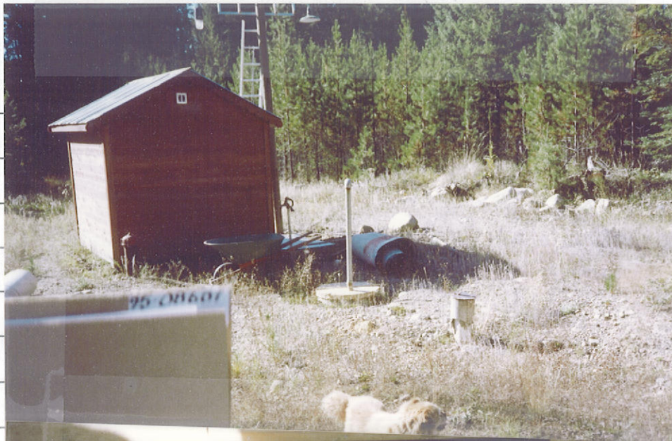
PUMP HOUSE WELL REF. IN FRONT OF BLDG. HOLDING TANK (CISTERN) IN FOREGROUND
