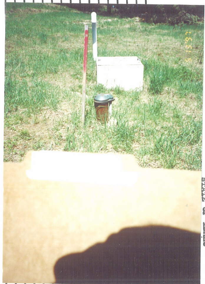
Well Head & Concrete Bunker
