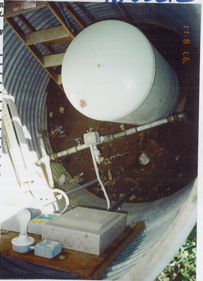
W.D. #1 - Well Head 6' Culvert with 3 Service Lines
