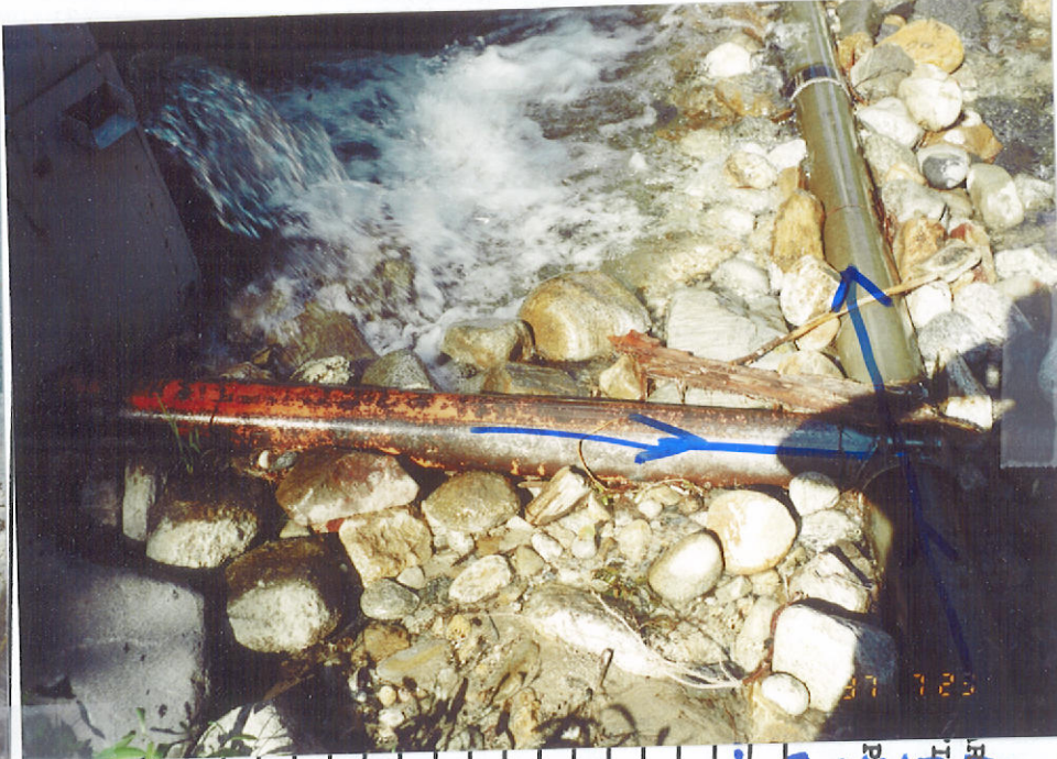
OVERDRAFT RETURN FLOW & CONNECTION OF P.D.#1 AND P.D.#2 SCREENED SETTLING TANK
