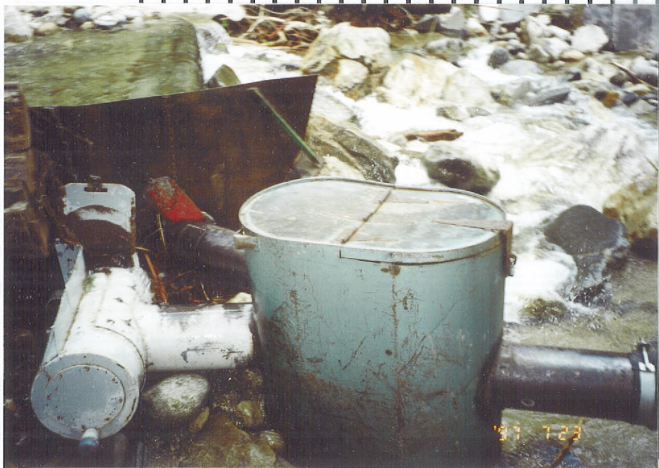
Generator & Bypass pipe P.D.#1 & Spillway
