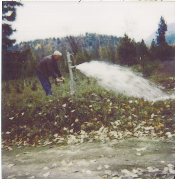
Fire Hydrant on 4000 Pack River Road
