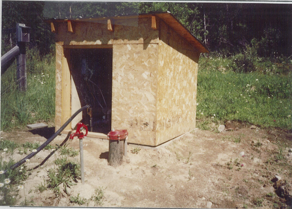
Well & "Pump" house
