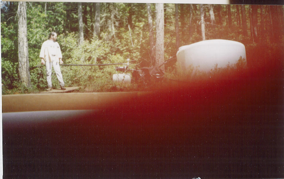
STORAGE CONTAINER w/ PUMP & MOTOR
