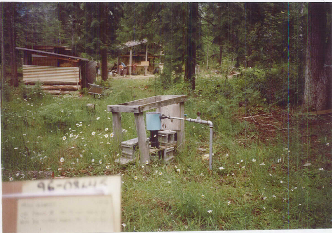
MR. MAHNKE GRAVITY FEED SYSTEM INTO THE HOUSE.
