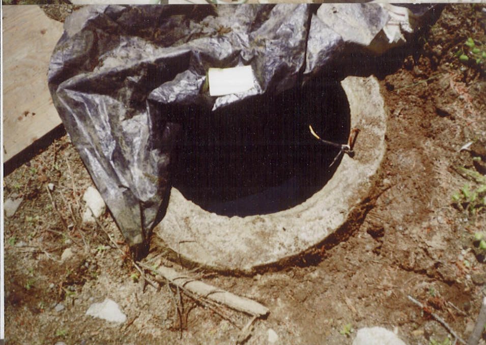
CISTERN w/ submersible ← pump
