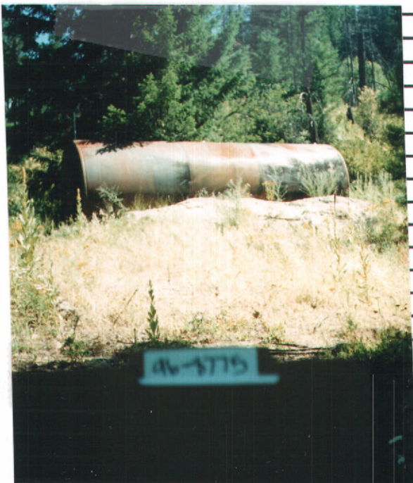
8000 gal Storage tank
