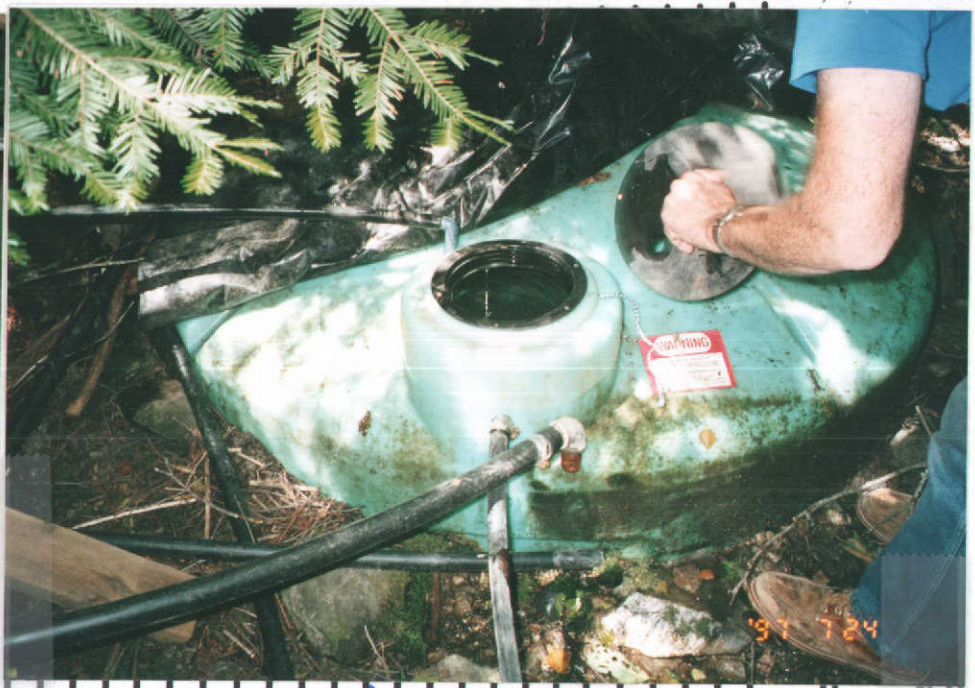
425 gallon holding Tank Hose and water supply hose
