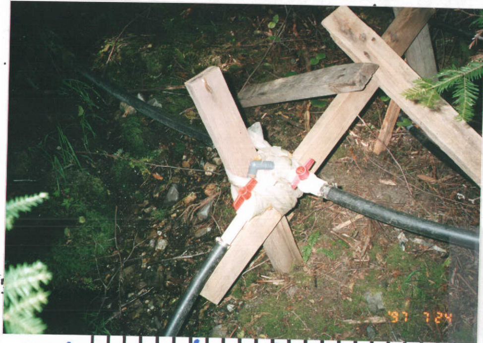
Valve System for Spring #2
