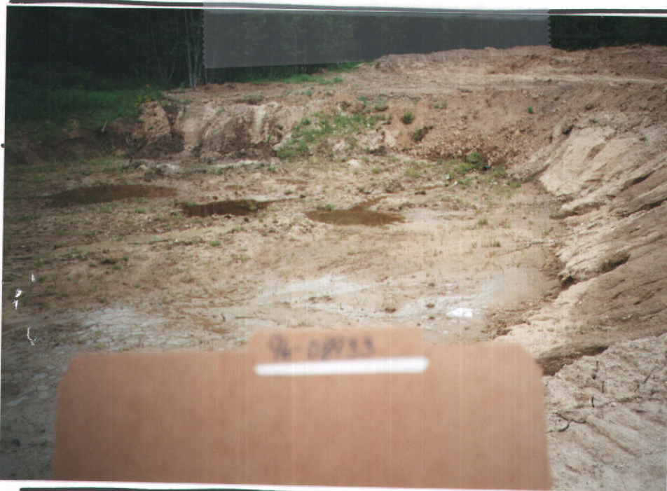
Bank around storage pond
