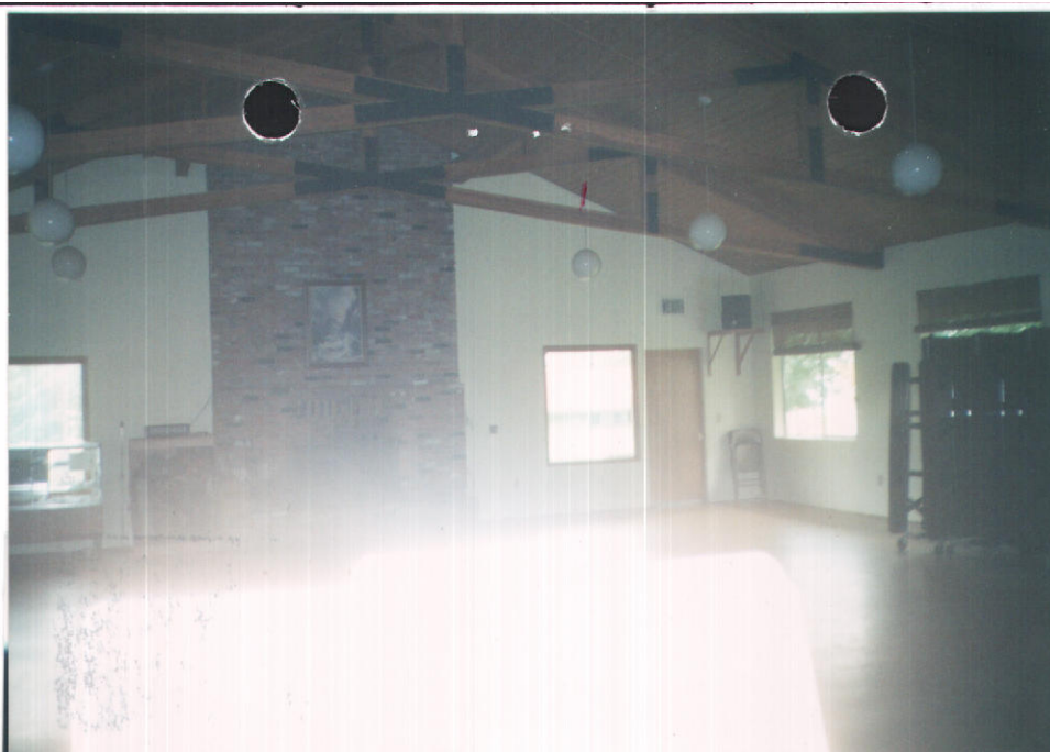
Dining Hall In building listed as office
