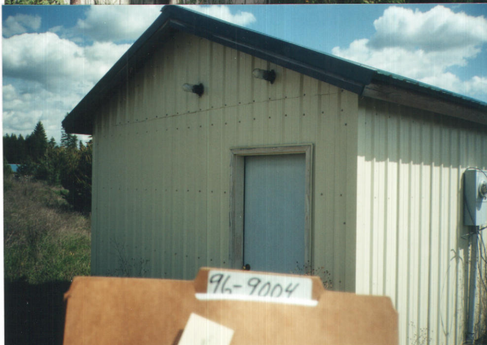
Pump House Sec 10
