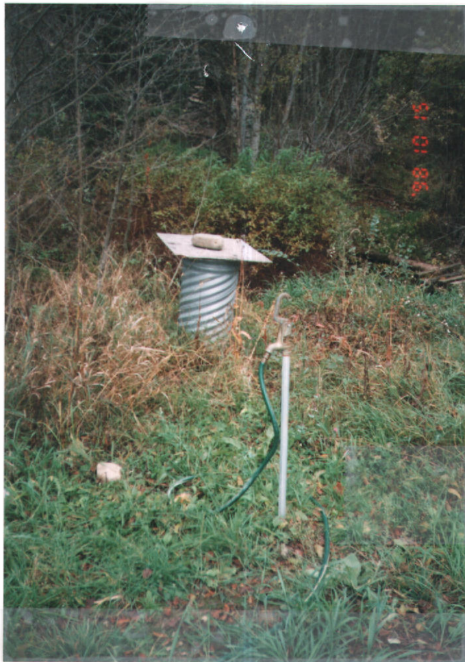
↑ SPRING & CULVERT CASING
