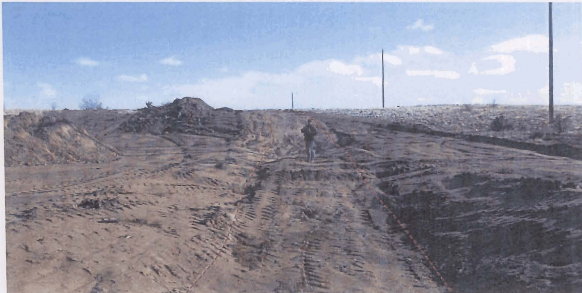
ABOVE: View from the excavated cutoff trench (red dashed lines) looking towards the left (south) abutment area.
