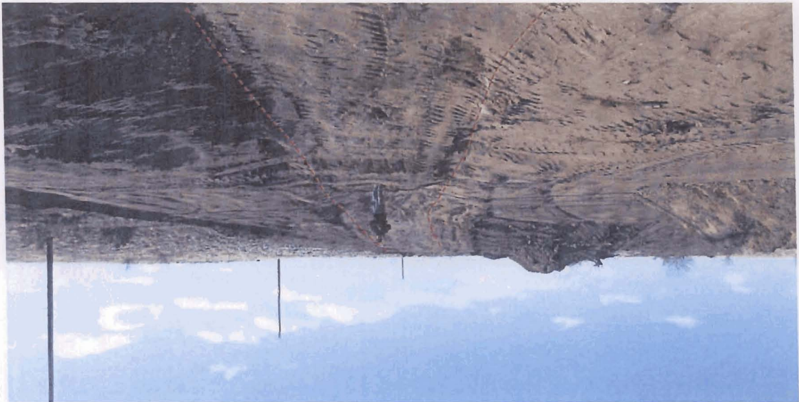
ABOVE: View from the excavated cutoff trench (red dashed lines) looking towards the left (south) abutment area. BELOW: View from the right (north) end of the dam site looking along the excavated cutoff trench (red dashed lines).
