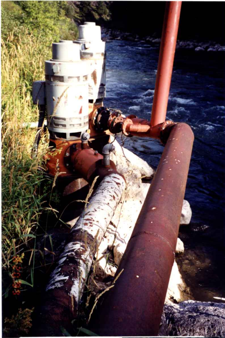
POINT OF DIVERSION (VIEW LOOKING UPSTREAM) TETON RIVER
