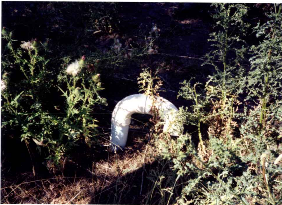
Point of diversion Siphon break looking North
