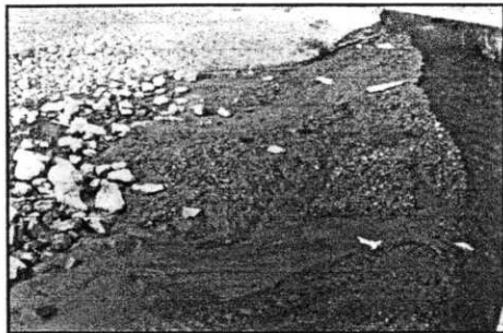
Close up of outflow area where sediment has built up over rock and is wet from previous high water flow
