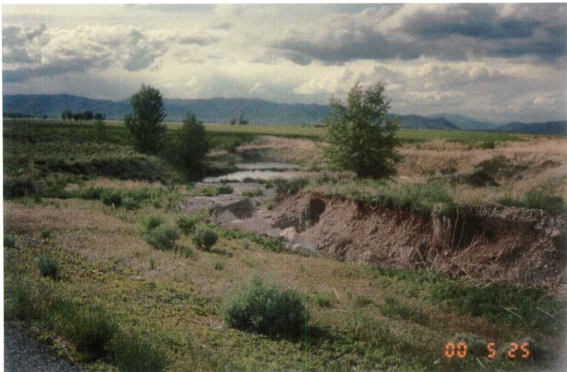
View looking at the existing gravel pit area North of Baseline Road. Notice high amount of erosion in the supply channel.
