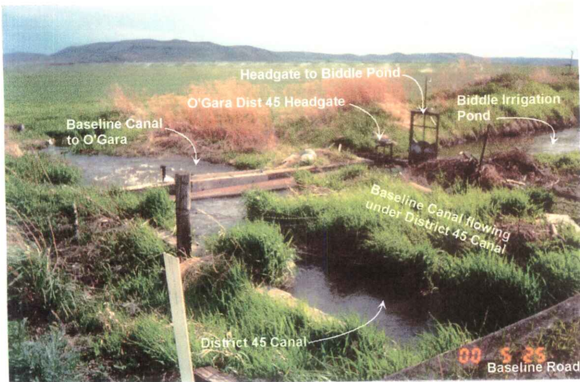
View looking south from Baseline Road showing confusing diversion works for the Baseline & Dist 45 canals. Both canals were running very high at the time of this photo.
