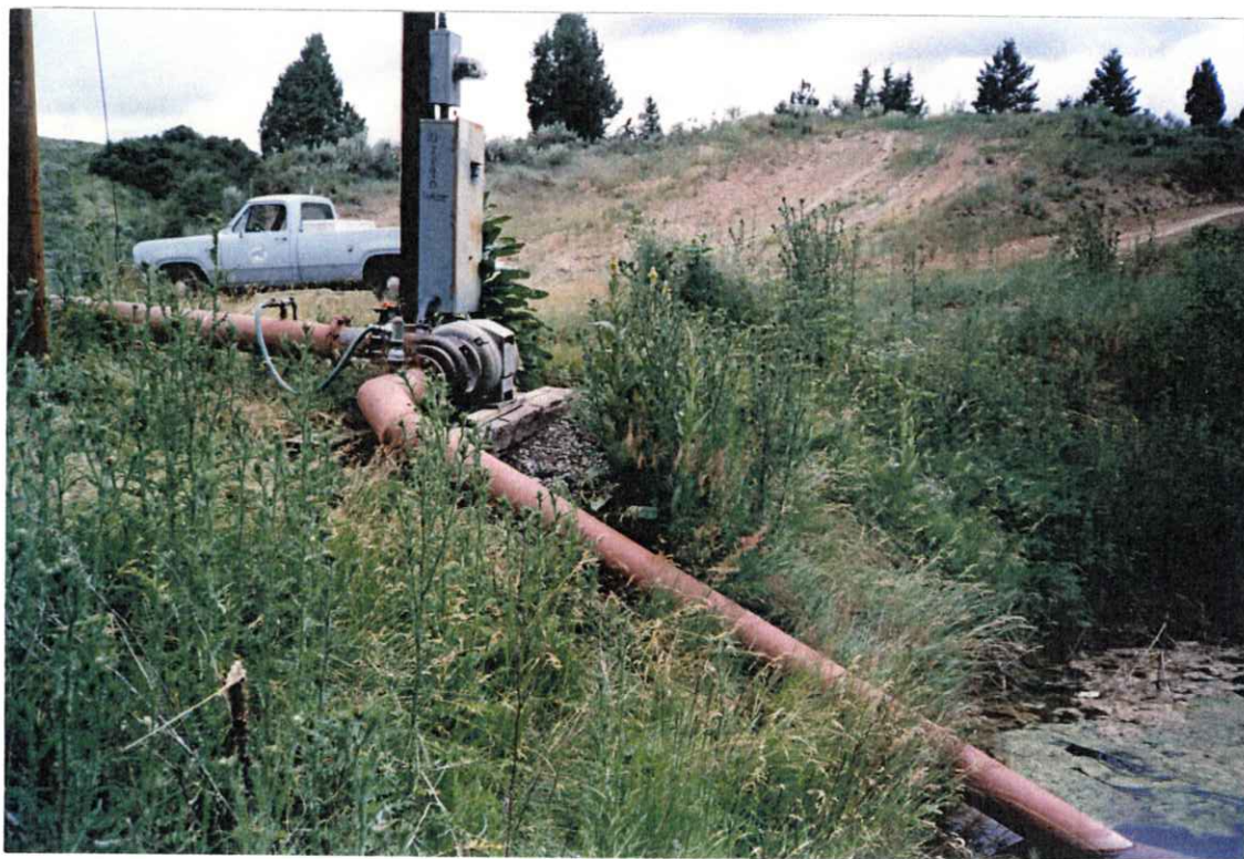
DIVERSION AT DIVERSION DAM ON UPPER RESERVOIR
