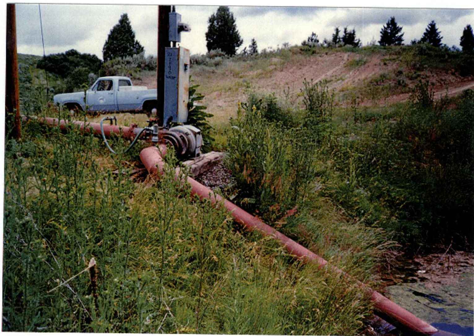
DIVERSION AT DIVERSION DAM ON UPPER RESERVOIR
