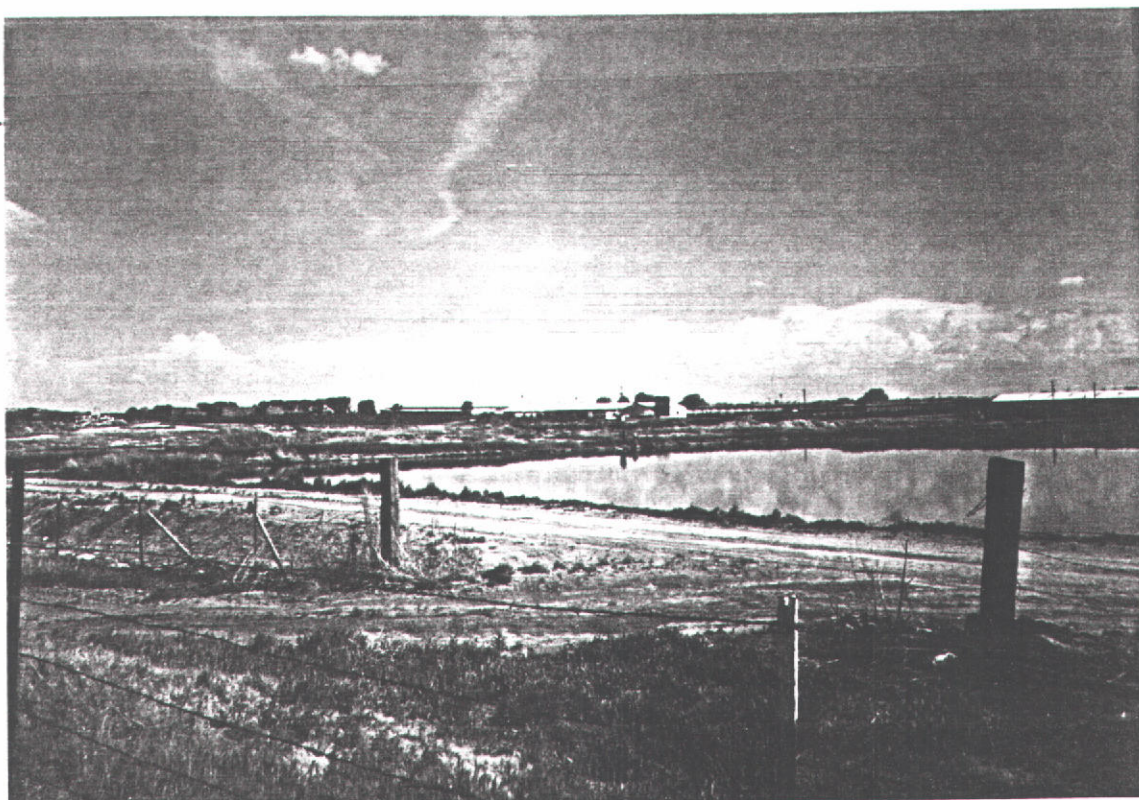
Dairy Lagoon + Pump South of Pivot (Looking SE)
