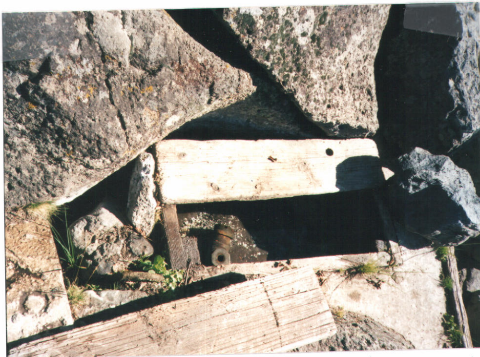
Spring box at Rock springs - Collection point for system
