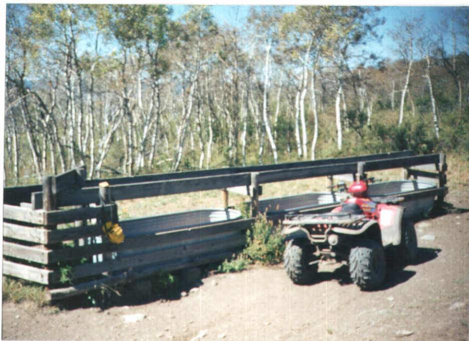
Looking SW at point of diversion #4 place of use
