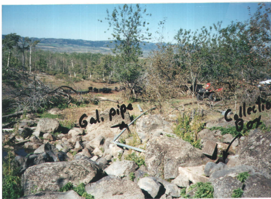
Looking West showing Collection Box and Permit #25-07350 the Gali. pipe going to System
