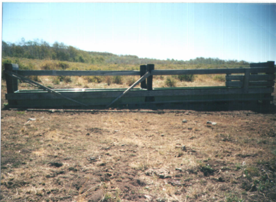
Looking East at point of diversion #3 place of use
