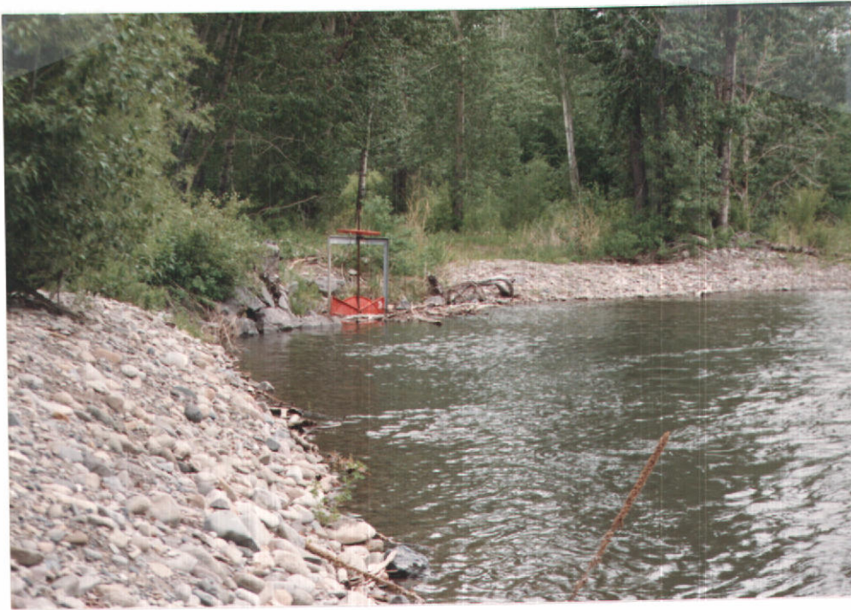
Headgate- Diversion R11A
