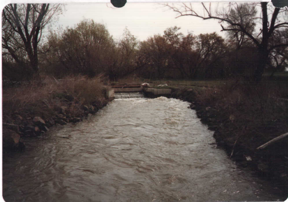
10' Radial gate Diversion
