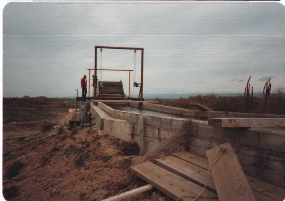
Forebat Canal at Penstock intake Looking downstream
