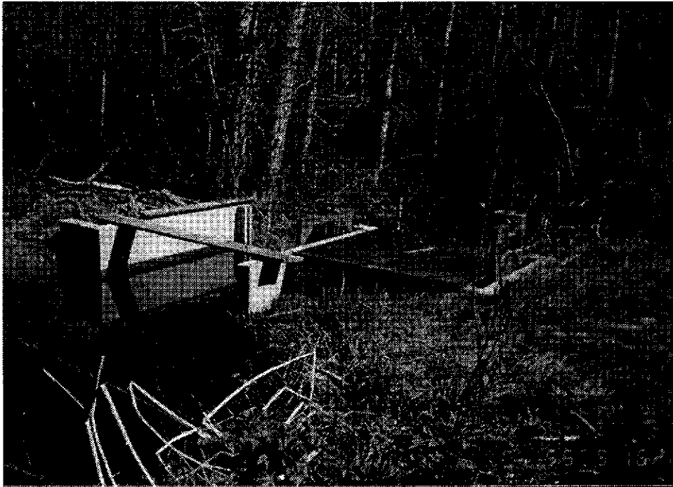
Figure 3. Submerged orifice diversion to Cliffside from Comstock Ditch.
