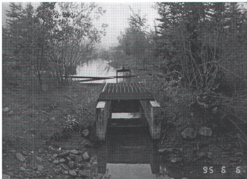
Figure 5. Broad-crested weir outlet to Comstock ditch from Cliffside to pond No. 6.
