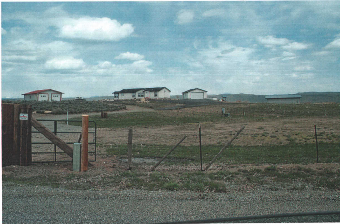
App 37-20718 Existing P/U Looking East From County Road By J E Stanton April 2002
