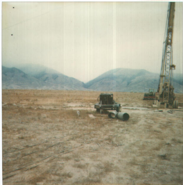
Well rig on well - 74-07290 3 October 1990 - no irrigation - no pump - no system. DMD
