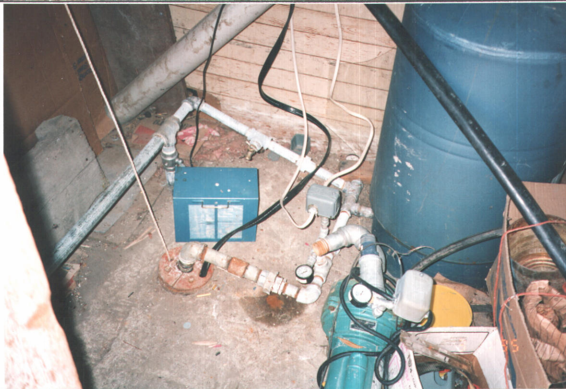
VIEW INSIDE OF WELL HOUSE
