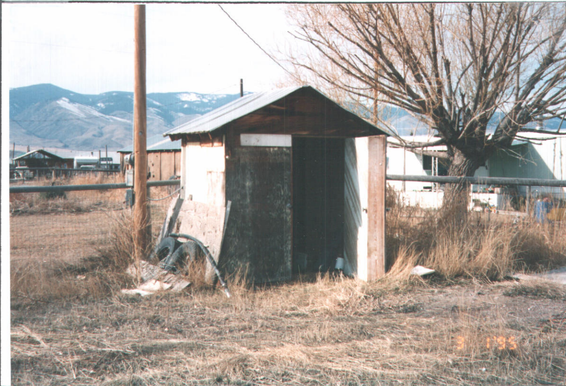
VIEW OF WELL HOUSE
