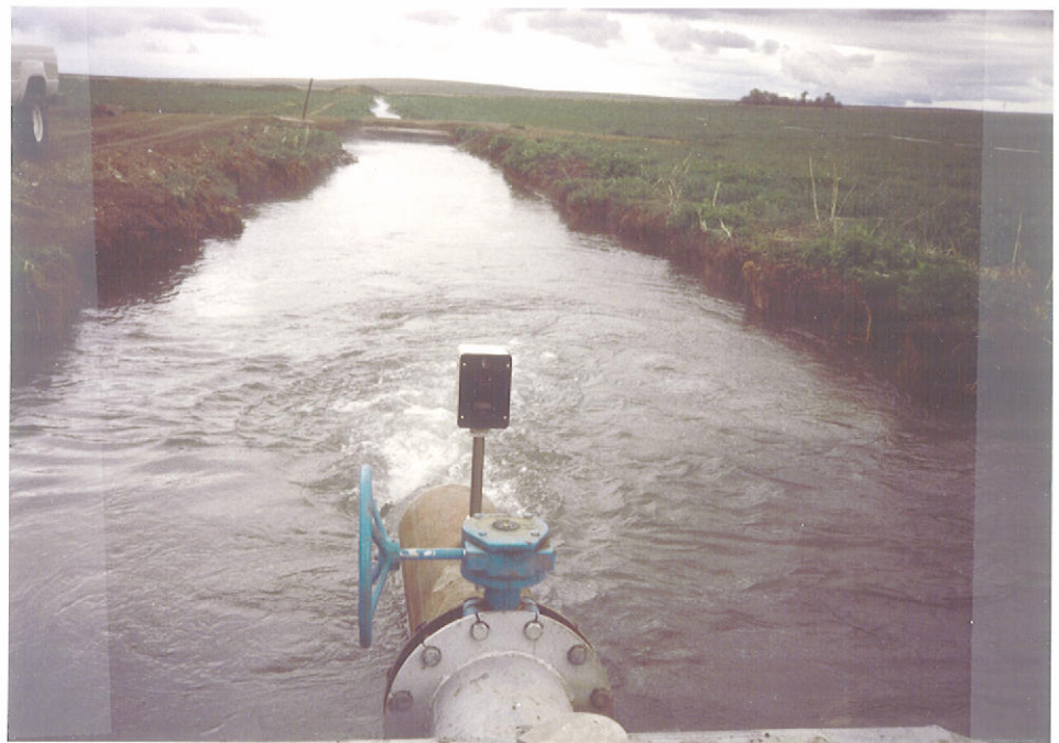
Ditch & P/U looking north. Note flow meter.
