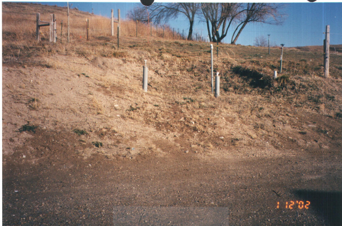
Buried storage tank + control valves
