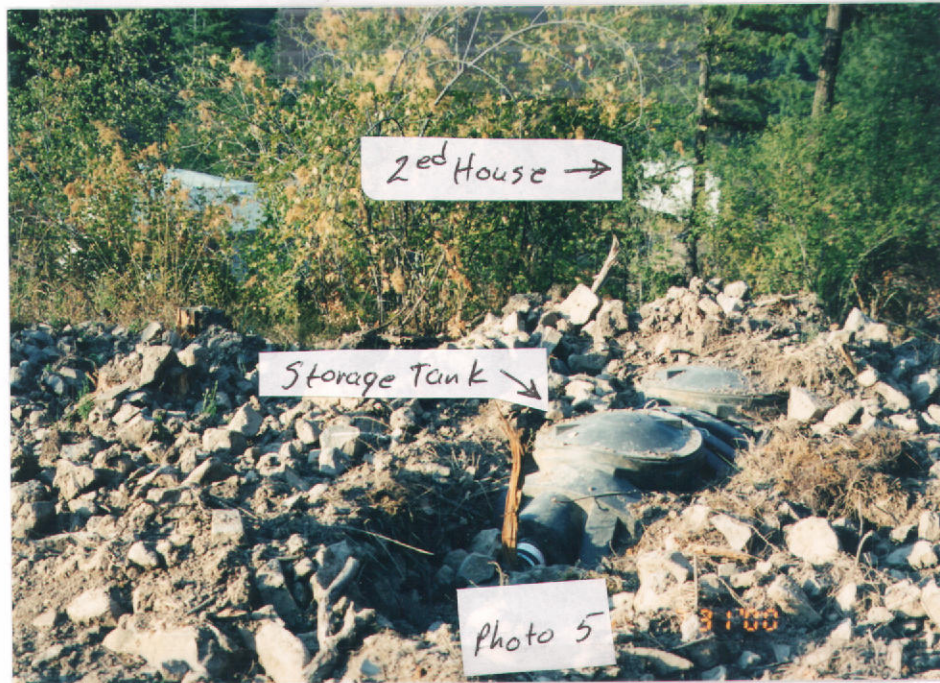
Photo 5. Showing 1000 gallon storage tank.
