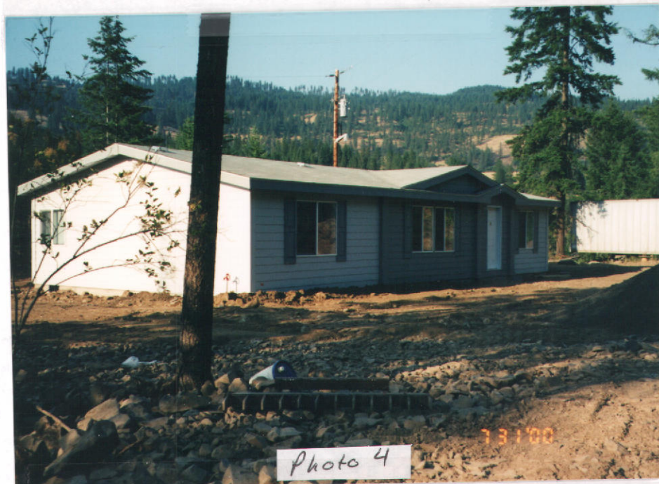
Photo 4. Showing house furthest from POD.
