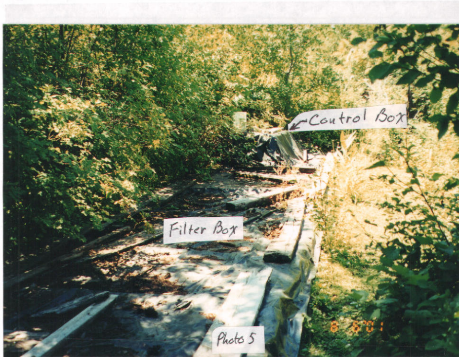
Photo 5. Showing filter box in relation to control box.
