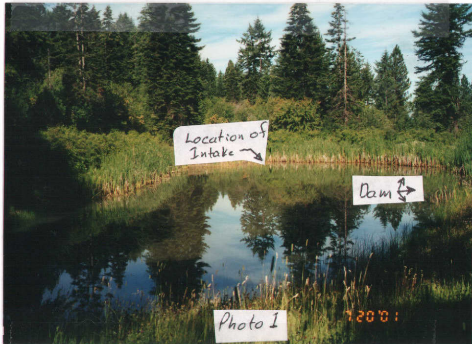
Photo 1. Showing pond and location of intake .
